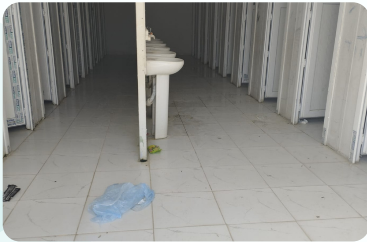
Comman Toilet Area
